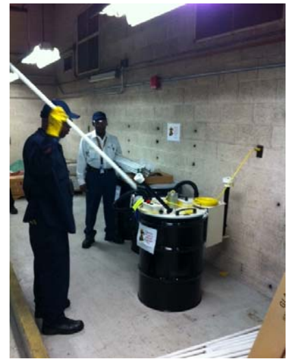
DOE Electrician Lovie Rose uses the bulb crusher while Building Engineer, Paul Young looks on.
